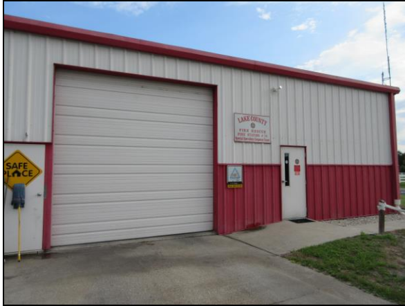
Station 76 in Yalaha, built in 1987 as a volunteer fire station, was not originally designed to house firefighters.
