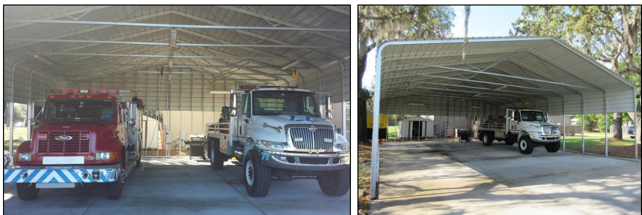
This open-sided metal structure does not provide adequate security for the fire vehicles.
